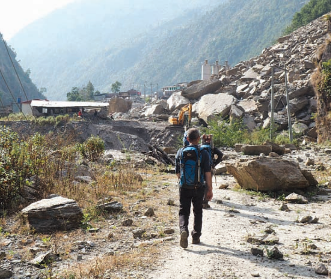
The final section of 'road'.
